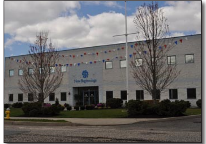
After years of planning and fundraising, the New Beginnings Community Center opened its doors recently.
